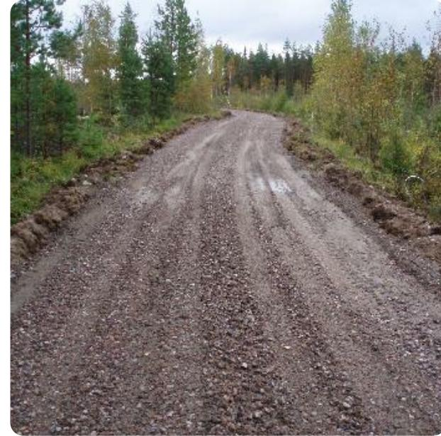
The ashes can be used in a road building among gravel. The use of ash from neighboring heat plants reduces the use of natural aggregates. The use of ash in the construction of the road has been limited, as it is currently subject to environmental permits.
